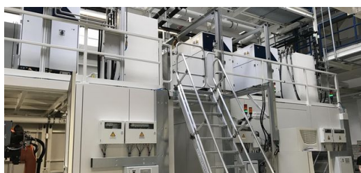
The CAMTRONIC section of the Mercedes-Benz plant in Berlin Marienfelde already fills more than one production hall. Production is organized as a linked flow line and is largely automated. Picture: Daimler AG
