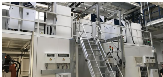
The CAMTRONIC section of the Mercedes-Benz plant in Berlin Marienfelde already fills more than one production hall. Production is organized as a linked flow line and is largely automated. Picture: Daimler AG
