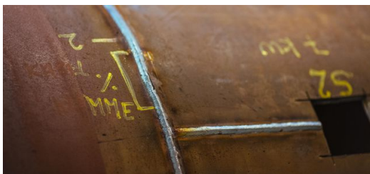
Welds up to 25 millimeters deep: Force Technology /LWT engineers use a 32-kilowatt laser to demonstrate laser hybrid welding processes for the maritime and the offshore wind turbine industries. Photo: Kasper Fladmoose
