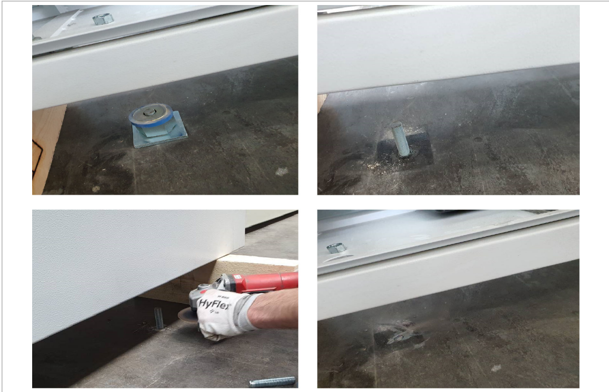
Severing the drop-in anchor
