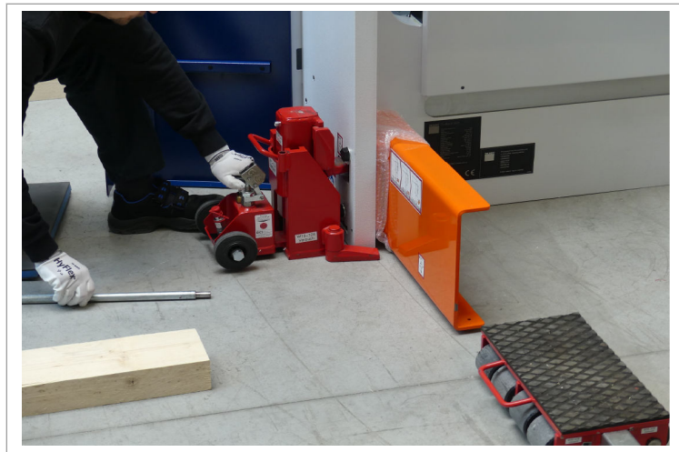
Lowering the machine onto the adjustable legs
