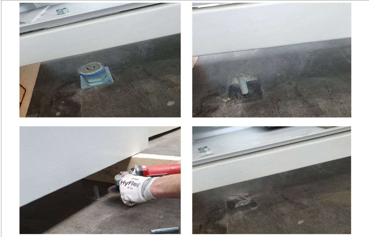
Severing the drop-in anchor
