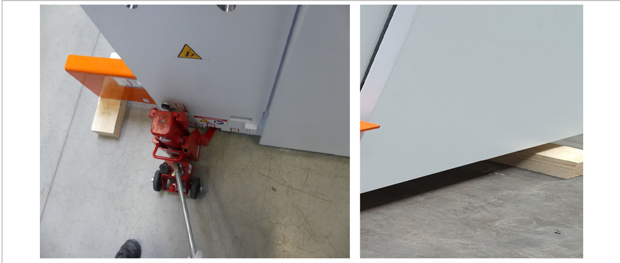
Lowering the right side of the machine to 80 mm
