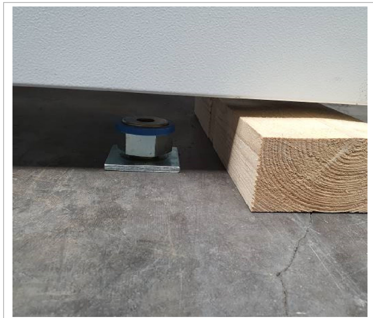
Aligning adjustable legs for drop-in anchors
