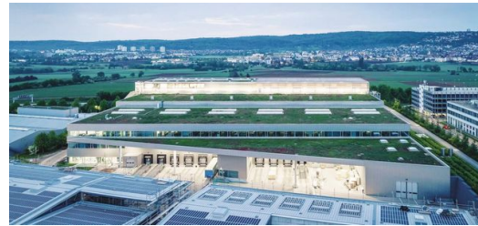
<p>Power from the rooftops: TRUMPF is steadily expanding its in-house generation of renewable energy through sources such as large photovoltaic systems.</p>
