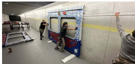
<p>The subway train art was put in place using brackets produced in-house on a TruMatic 7000.</p>
